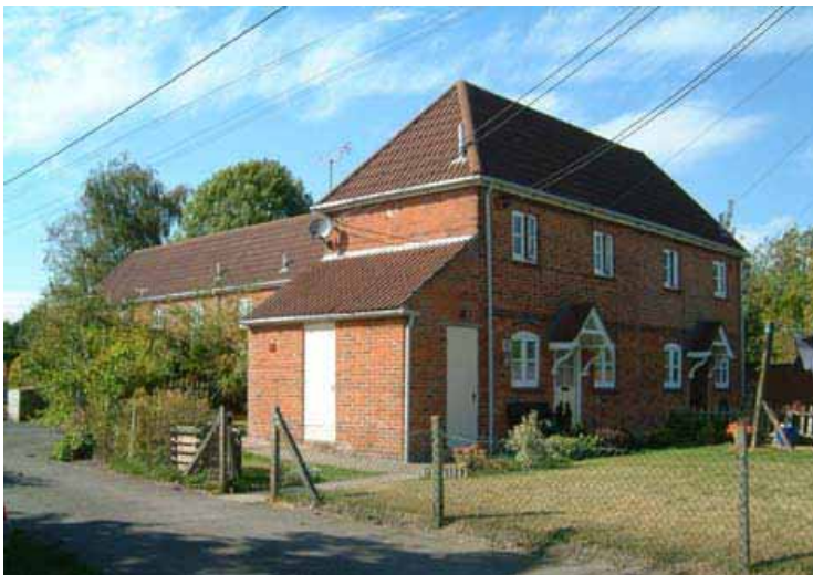
Early 19th century. 'The Barracks' once with chimneys and thatched.
