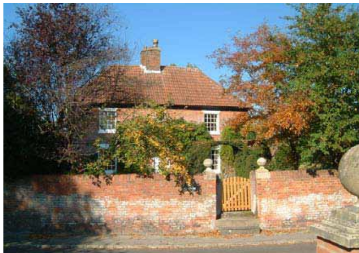
The Old Manor fronting onto one of the few roadside footways in the village
