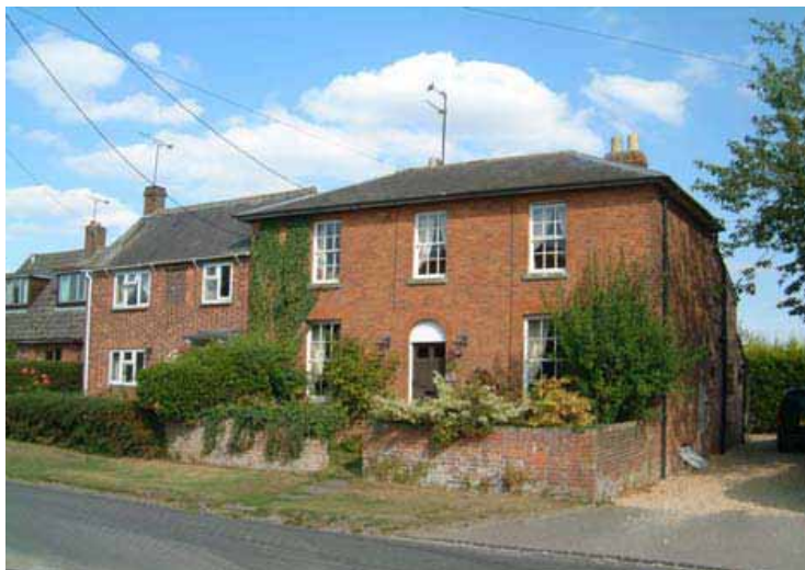
Nos.30 and 28 The Street. An early 19th century cottage attached to a mid 19th century villa
